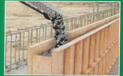
Concrete forming and base for laminating.
